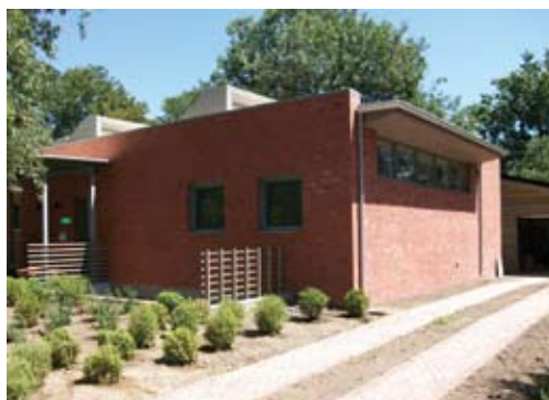
Logan Wiggins House 3, pictured here, is a zero net energy home in Boulder, Colorado. It was designed by Jim Logan Architects to be carbon-neutral and to produce more energy than it consumes. Credit: jlogan.com
